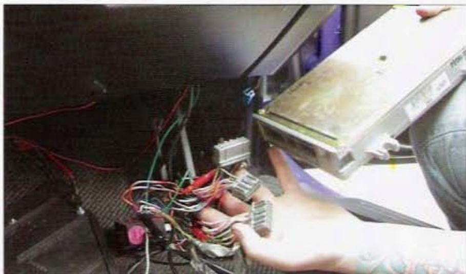
OBD wiring conversions are time consuming and tedious. You need to cut off each one of these wires entering the ECU of this late-model Integra and solder them into place on the Civic or CRX of choice.
